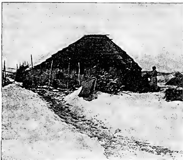
HOUSE IN DEMOLITION: SHIRAOI.
